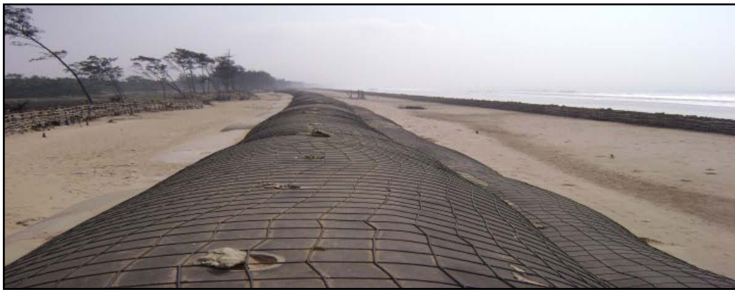
Fig 8. Coastal Erosion Management Steps ( Geo-Tube Concept) at Sankarpur
