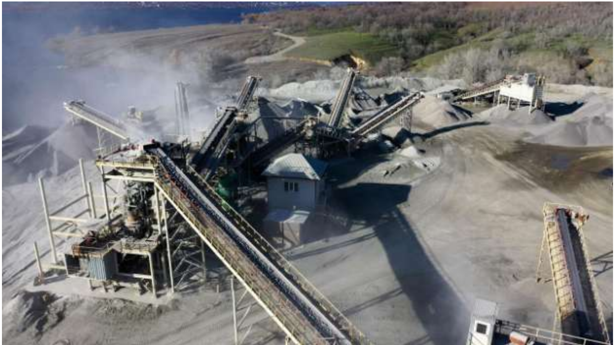
Figure 1.1: A minerals processing plant and an overview of the conveying system between crushers, screens and storage units.
