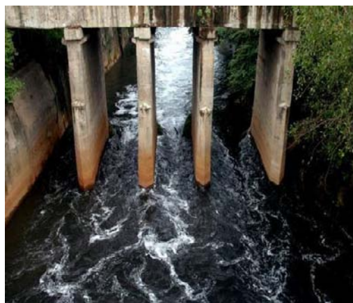
Figure 2: Dirty water in the Drain
