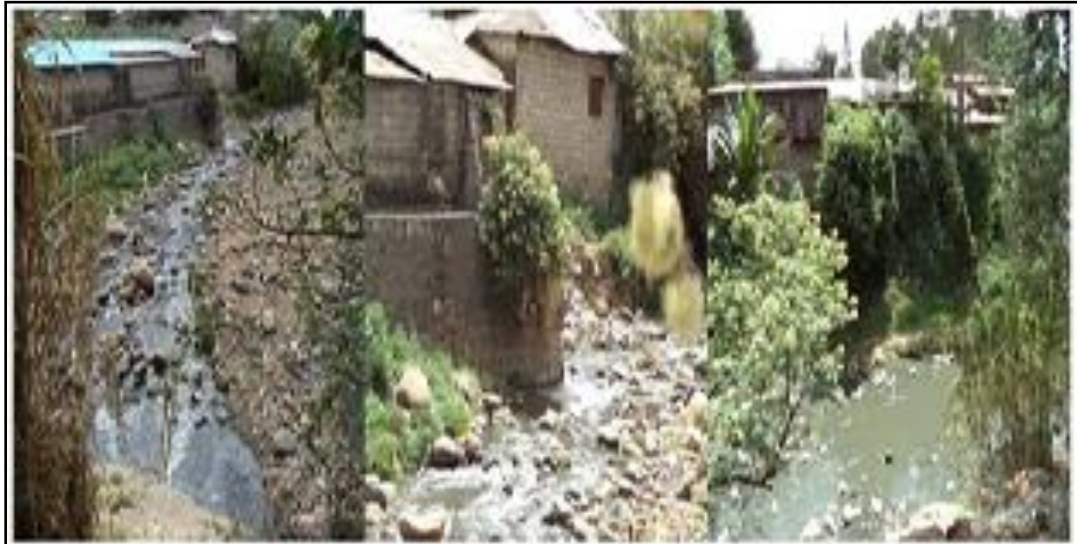
Figure 21: Stream encroachment by Buildings in the study area (Bole sub city-Addis Ababa)
