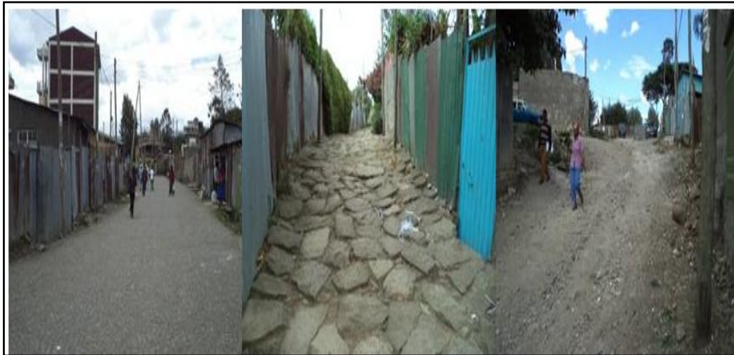
Figure 8: Existing road surface of the study area (Bole sub city-Addis Ababa)
